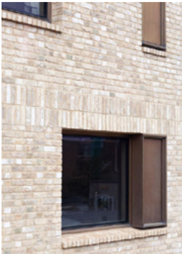
Selected brick or brick panel system with buff tone colour, raked mortar joint, varied mortar colour.
