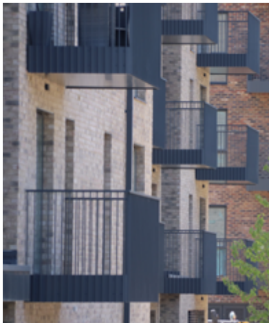
Projecting Balconies with Selected PPC vertical balustrades
