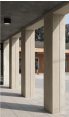
Pre-cast composite stone cladding panel system in pale stone colour.
